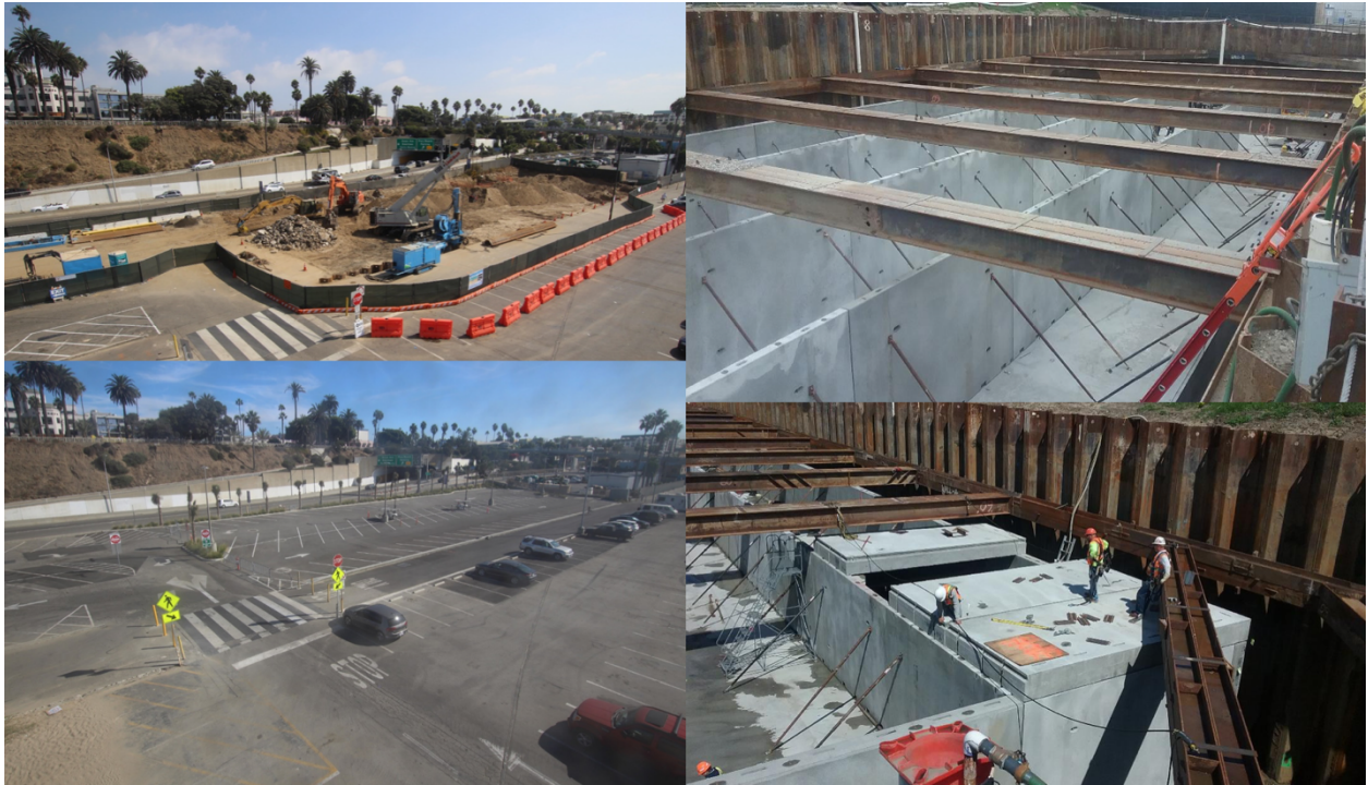
Clockwise from top left: excavation for storage reservoir; construction of pre-cast walls for storage reservoir; installation of pre-cast walls and top panels for storage reservoir; completed parking lot on top of the storage reservoir. [Photos courtesy of the City of Santa Monica's Public Works Department]
