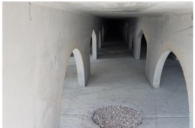
Albion Riverside Park (Four Photos Above)
