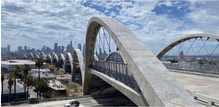
Photo courtesy of Skanska-Stacy and Witbeck (SSW)
