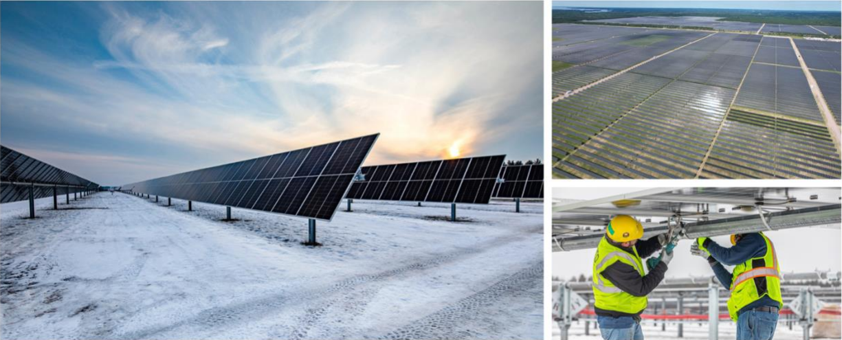
Bottom right: Securing PV panels to the tracker system during construction.
