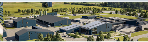
Bull Run Filtration Facility, Portland, OR, Envision Platinum (v3) 2025
