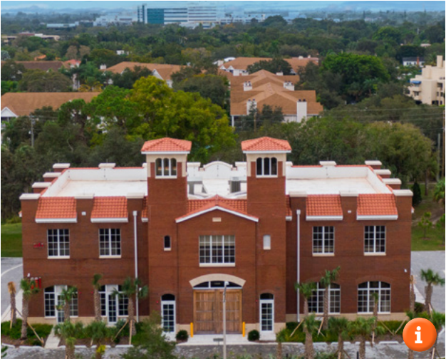
City of Sarasota's Lift Station 87, Sarasota, Florida, USA, Envision Silver 2025
