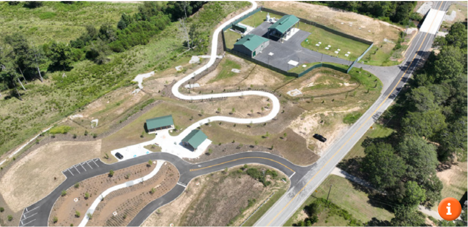
Eastern Regional Infrastructure Project, Gwinnett County, GA, USA, Envision Silver 2024
