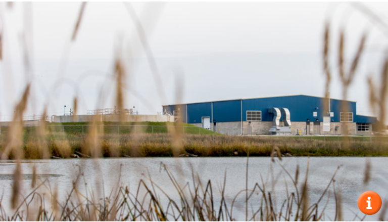
Grand Bend Area Wastewater Treatment Facility, Lambton Shores, Ontario, CAN, Envision Platinum 2015
