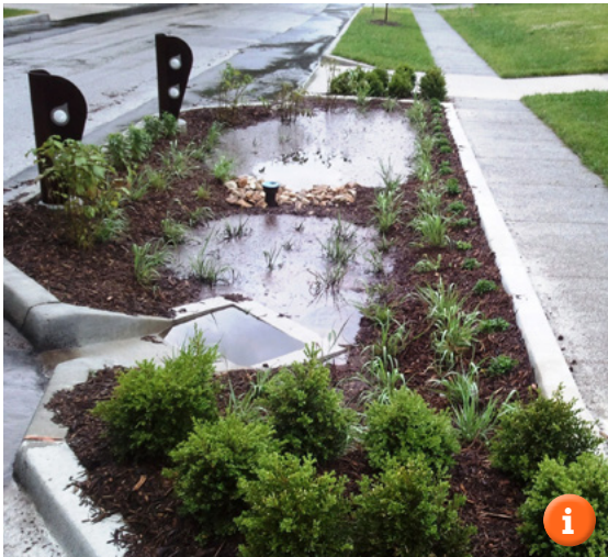
Middle Blue River Green Infrastructure Project, Kansas City, MO, USA, Envision Platinum 2016
